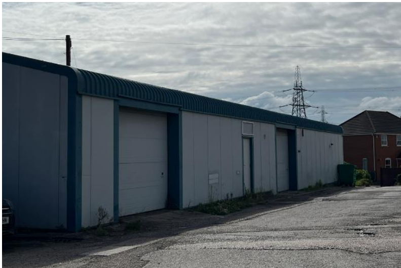
Figure 23 - Old Pill Farm Industrial Estate
